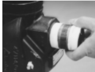
Step 3: Install the 2" (50 mm) nipple (Item #4) in the Series 717R valve body.
