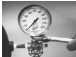
Step 7: Install the water pressure gauge (Item #3).
