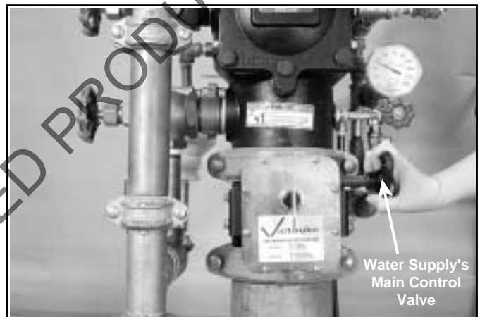
27. Open water supply's main control valves slowly until a steady flow of water flows from the open water supply main drain valve.
