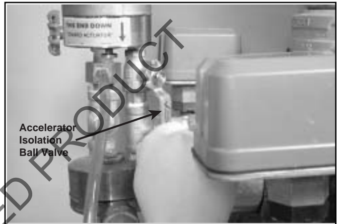
20a. Open isolation ball valve to accelerator.
