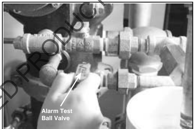
9. Confirm that the alarm test ball valve is closed.
