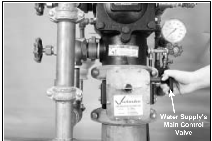
4. Close water supply's main control valve.
