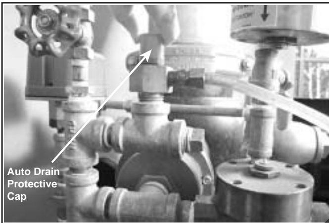
23. Remove protective cap from Series 749 Auto Drain.
