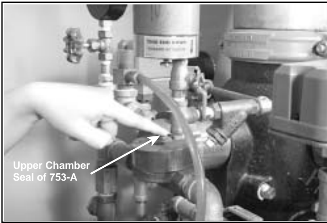
17a. While system is charging, it may be necessary to push down on upper chamber seal of Series 753-A Dry Actuator.
