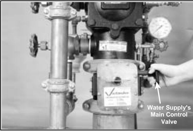
9. Close water supply's main control valve.
