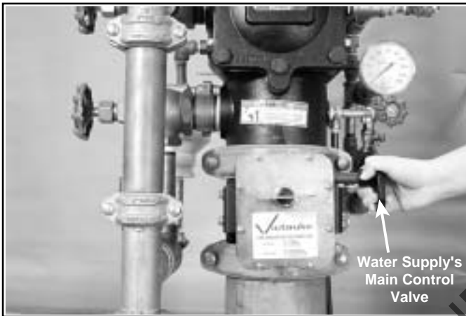
4. Close water supply's main control valve.
