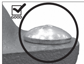
OVAL NECK OF BOLT SEATED PROPERLY
