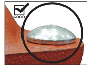
OVAL NECK OF BOLT SEATED PROPERLY OVAL NECK OF BOLT NOT SEATED PROPERLY
