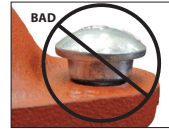
OVAL NECK OF BOLT NOT SEATED PROPERLY
