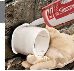
Caulk wall opening.
