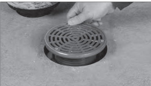
Install Finish Fixture
