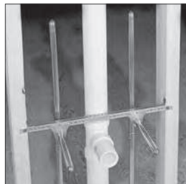
Test-ready stub outs and air chambers, with only ONE solder joint needed.
