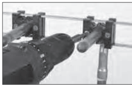
Install stub out and tighten screws on blocks.
