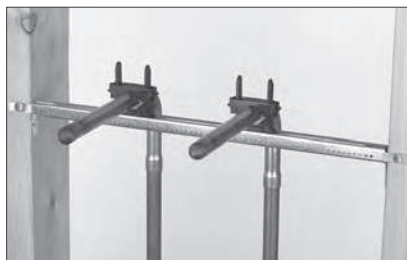
Place tube inside clamps and cinch the bridge down evenly over posts to secure.
