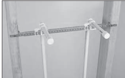
Use Edge Clamps with galvanized models.
