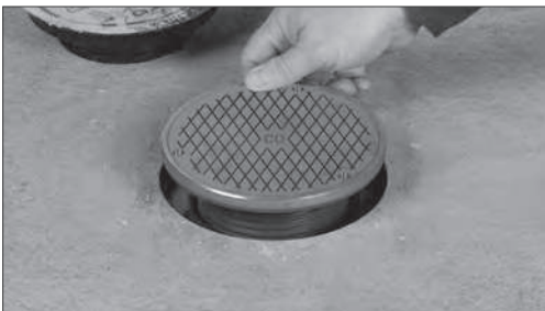
Install Finish Fixture
