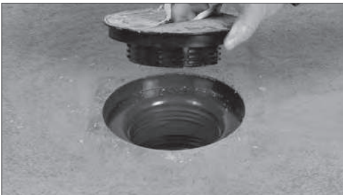
Remove Coring Plug
