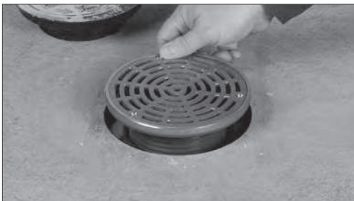
Install Finish Fixture
