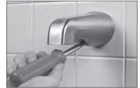
Tightens firm and flush to the finished wall.
