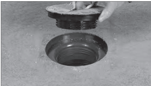
Remove Coring Plug
