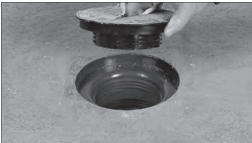
Remove Coring Plug
