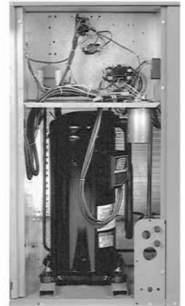
Compressor Access (SLKA-A036, 042, 048, 060, and 072 Models)
