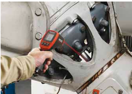
Diagnose temperature of wear parts for preventive plant maintenance
