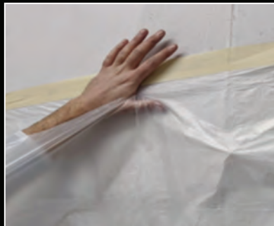
Remove dirty layer by sliding hand through perforation at top to reveal another clean layer.
