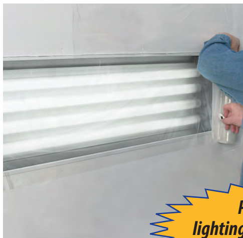
Finishing up at end of glass and cutting with SNIPPET KNIFE or razor blade.
