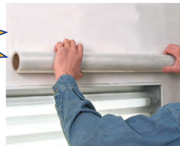
Roll down film against wall smoothing as you go to the top of lightbox.
