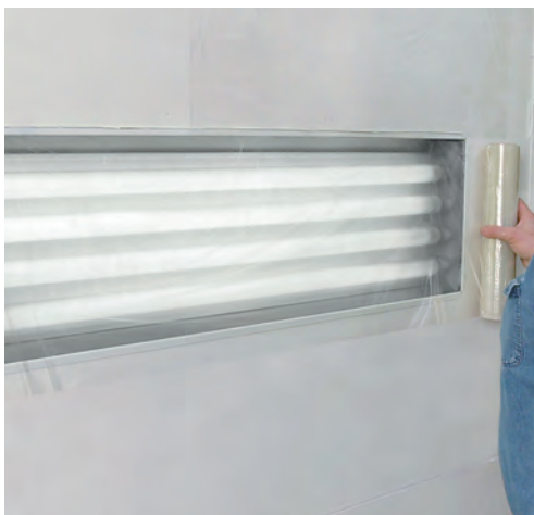
Finishing up at end of glass and cutting with SNIPPET KNIFE or razor blade.
