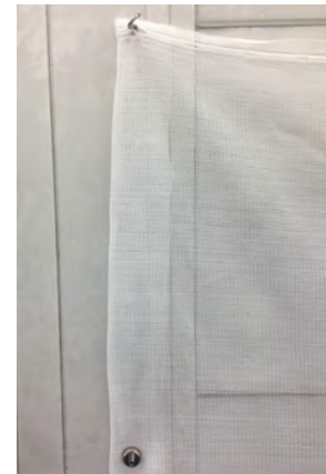
After cutting netting fold over and secure with magnets for a clean edge.
