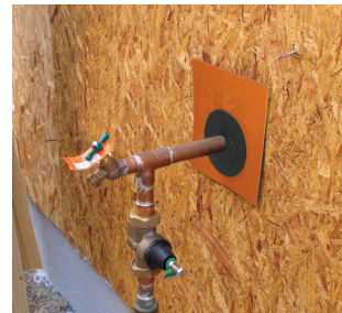
Oatey Sideflash creates a constant seal for superior protection.
