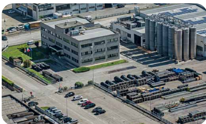
Production Facility - Castel Guelfo di Bologna (BO)
