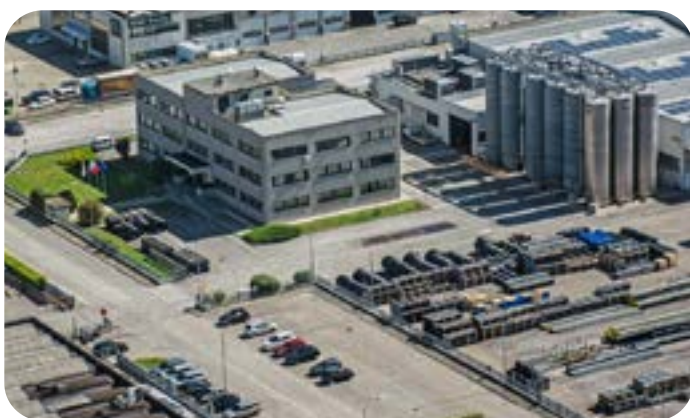
Production Facility - Castel Guelfo di Bologna (BO)
