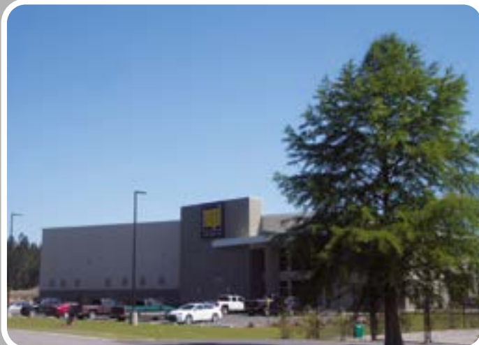
Production, Operations & Administration Center - NUPI AMERICAS INC. - Early Branch (SC)
