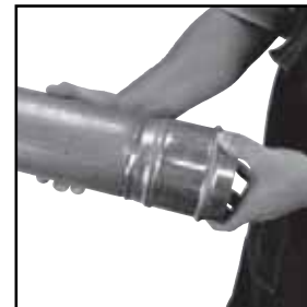
Figure 9: Inspection of final crimp
