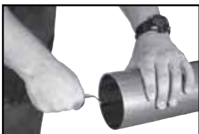
Figure 3: Deburr inside diameter deburring tool
