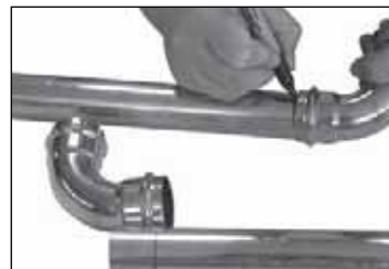
Figure 3 — Inserting the tube to proper depth
