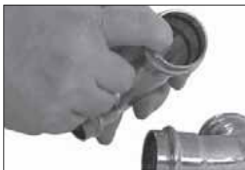
Figure 2 — Check for EPDM Seal
