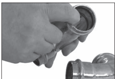
Figure 2 — Check for EPDM Seal
