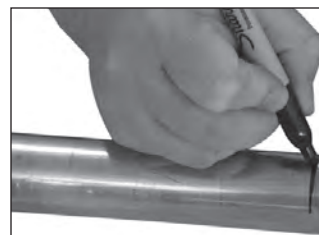
Figure 3 — Marking for Insertion Depth
