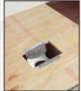
Mount SureGrip support plate.
