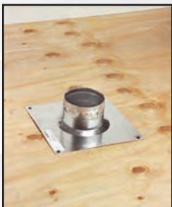
Push pipe through vent support.
