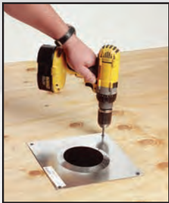
Mount SureGrip support plate.
