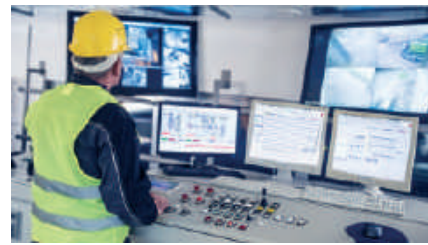
Remote Control Room
