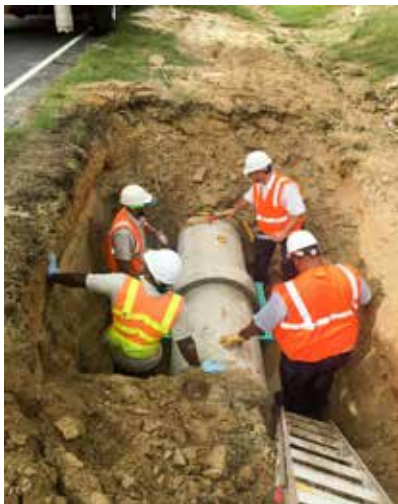
JCM 114 Mechanical Joint Bell Repair Sleeve installed over problematic leaking Asbestos Cement Coupling
