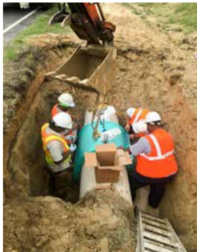
JCM 114 Mechanical Joint Bell Repair Sleeve installed over problematic leaking Asbestos Cement Coupling
