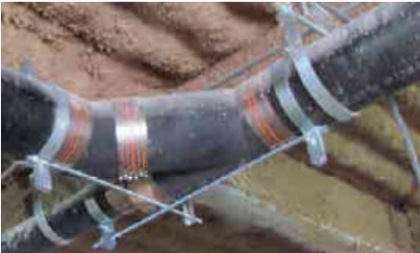
No-Hub Fitting Restraint
