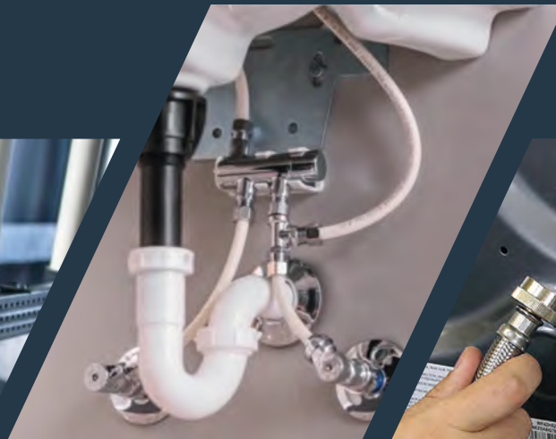
Valves and Supply Stops
