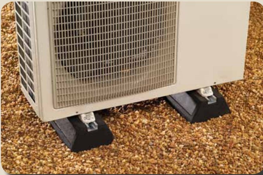
Hef-T-Foot™ – Rooftop/Ground Mount Installation
