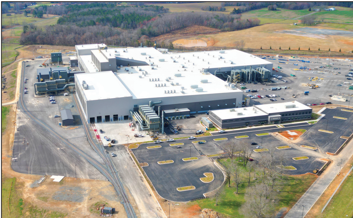
Charlotte Pipe and Foundry Company's new foundry at Oakboro, NC
