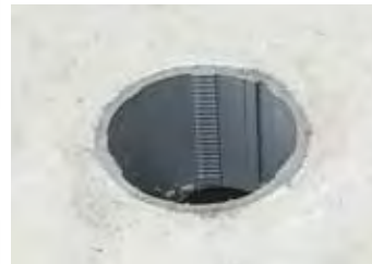
Cut box top level with concrete
