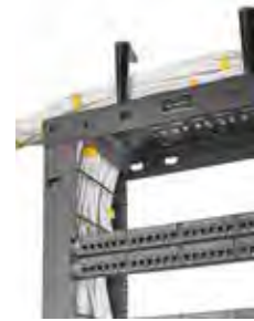
Wire Gates Installed
