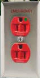
Critical care spaces in a healthcare facility require 100% reliable power and data connections without interruptions. These demanding 24/7 environments encounter significant abuse such as abrupt plug removal and numerous insertions, being impacted with carts, beds and gurneys, exposure to harsh cleaning disinfectants—all of which can contribute to damage.
