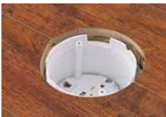
Wire devices into box
