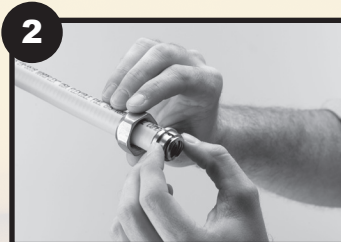
2 Slide nut over tubing, place retainer ring leaving one corrugation exposed.
