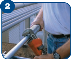
2 With a wrench, tighten the gland nut to compress the Teflon® packing, creating a raintight seal around the conduit.
