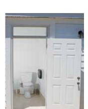
Bathroom equipped with Saniaccess3 macerator which discharges the waste through a small diameter pipe into the holding tank.
