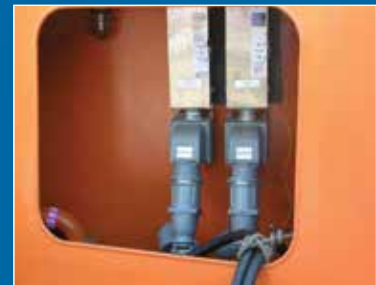
200A MaxGard® inlets with disconnects
