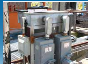
200A MaxGard® interlocks in parallel
