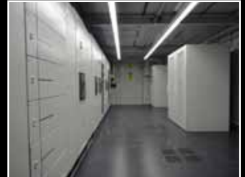
LER Extend with Power Distribution / UPS
