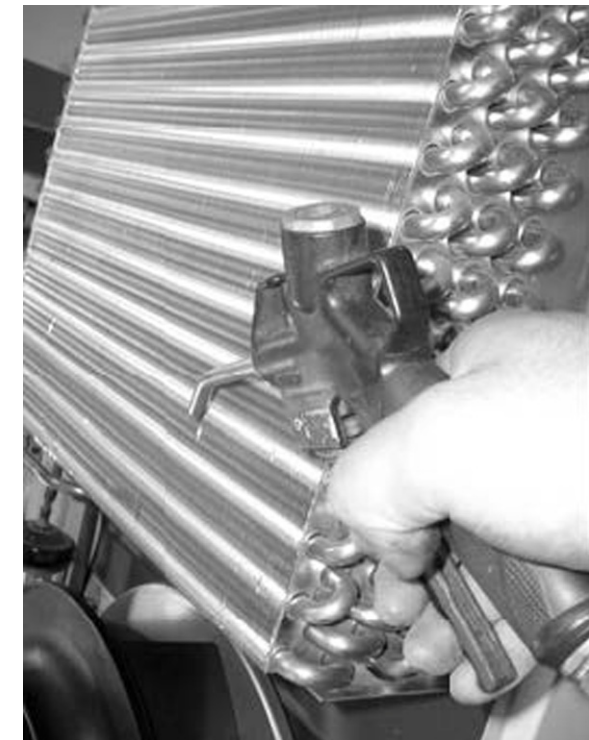
Fig. 30: Clean out the heat exchanger coil and compressor chamber using compressed air
