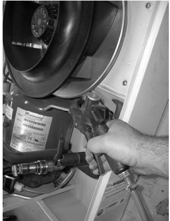
Fig. 31: Clean out the heat exchanger coil and compressor chamber using compressed air
