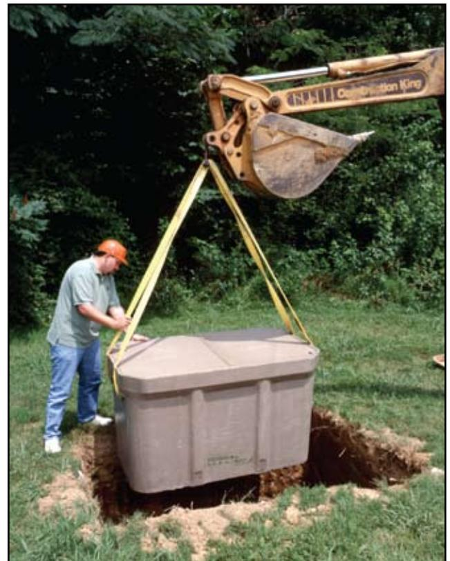
QUAZITE® enclosures are lightweight for easy installation.
