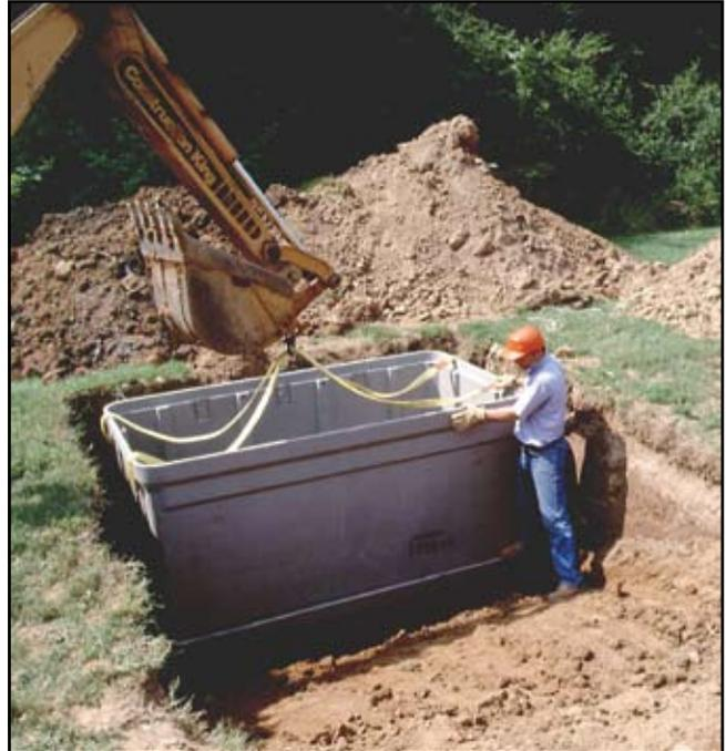
The strong polymer concrete construction allows QUAZITE<sup>®</sup> enclosures to be stacked for even greater depths.
