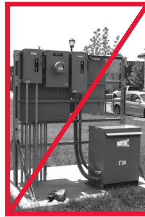
Strut and backboard
