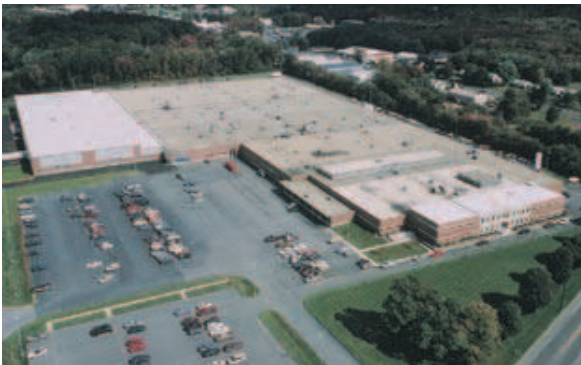
LENOX® ISO 9001 certified facility in East Longmeadow, Mass., U.S.A.
