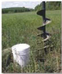
Prepare hole for pole
