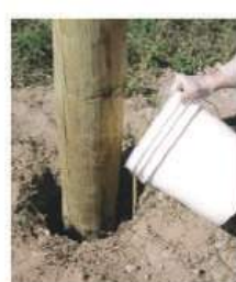
Pour mixture into prepared hole with pole
