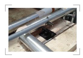
Roof Top Blox are designed specifically as roof supports to be used on commercial roof piping support and platform support applications.
