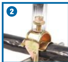
2 Using a power tool fitted with a ¾" (16mm) socket, tighten lock nut...
