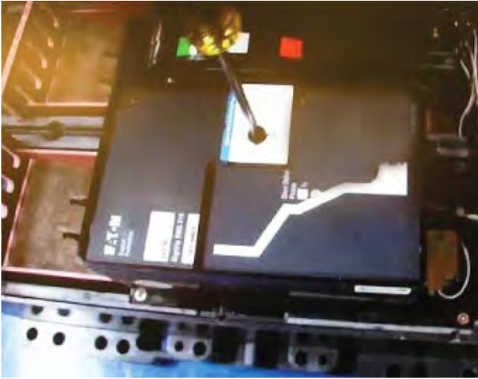
Figure 3. Unlocking the Rating Plug.
