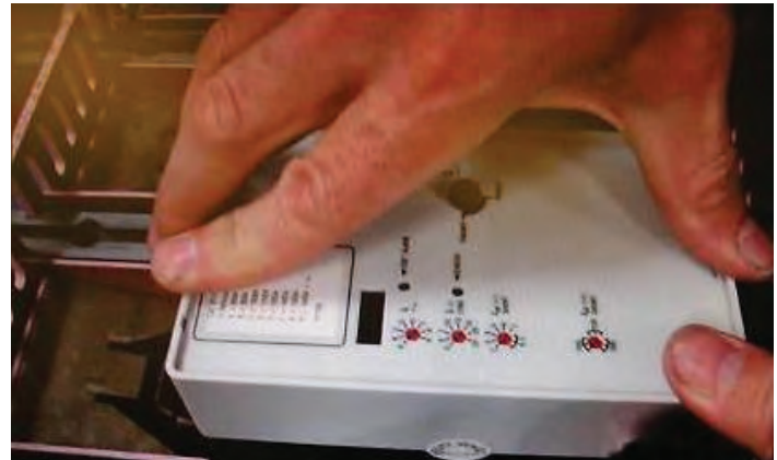
Figure 15. Installing the RG 310+ Trip Unit.
