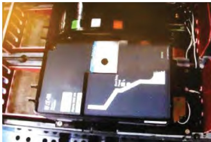
Figure 2. Trip Unit to Be Removed.
