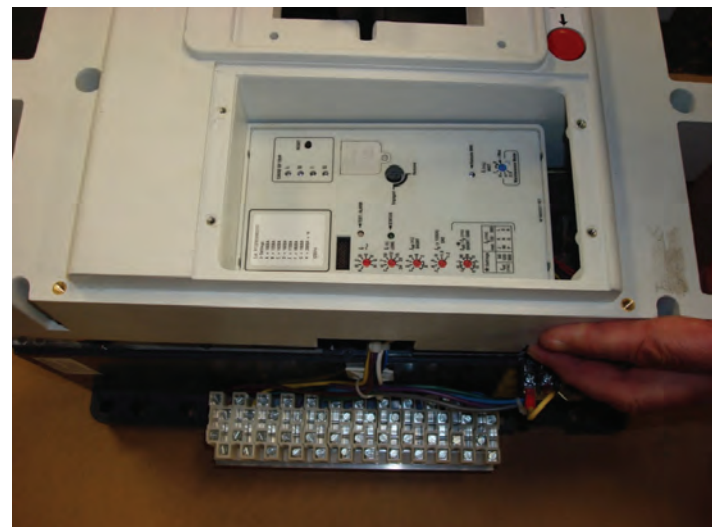
Figure 20. Replacing the Breaker Cover.
