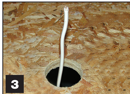
Figure 3 - Pull NM Cable through floor.
