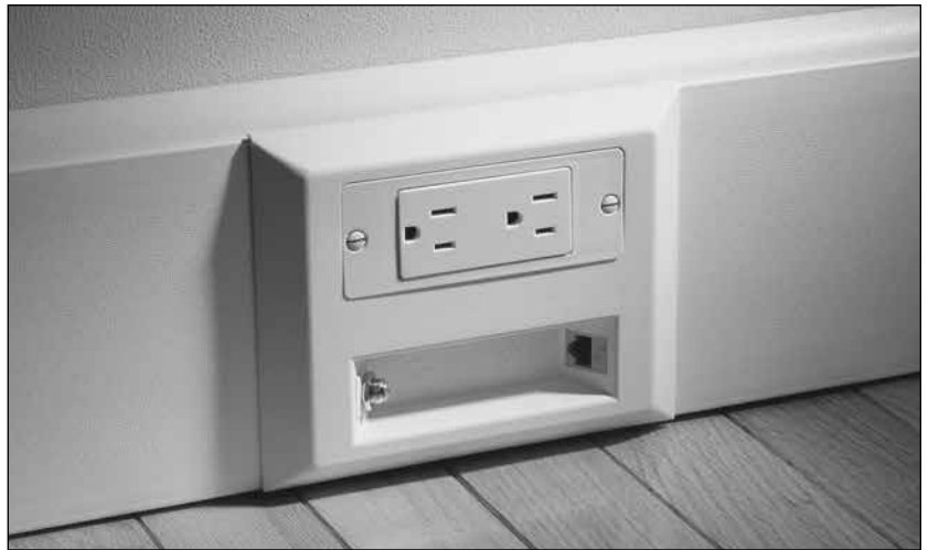
Access 5000 Series Raceway installed as baseboard.
