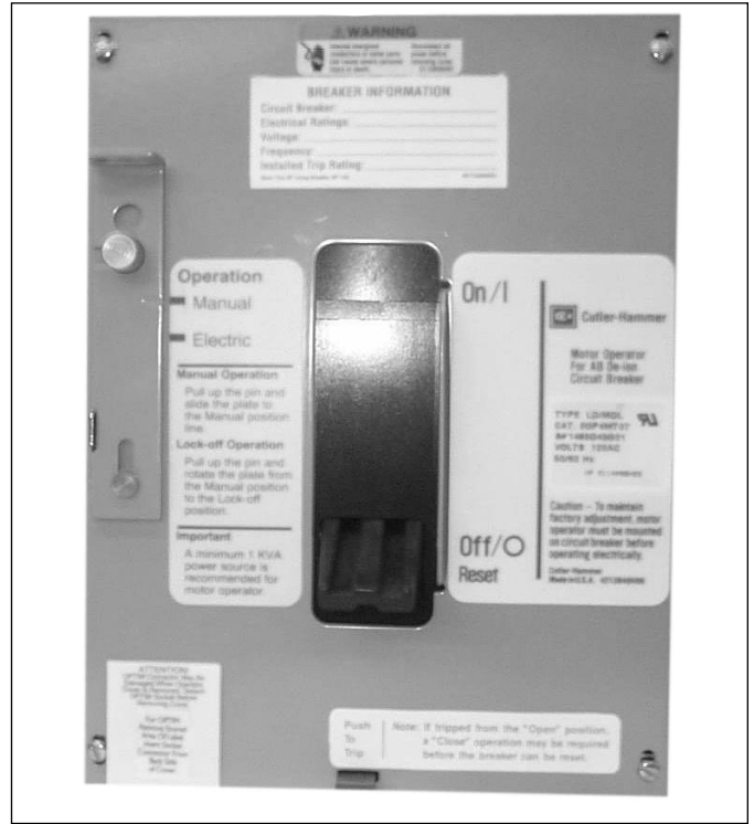
Figure 3-3 Motor Operator in Manual Position
