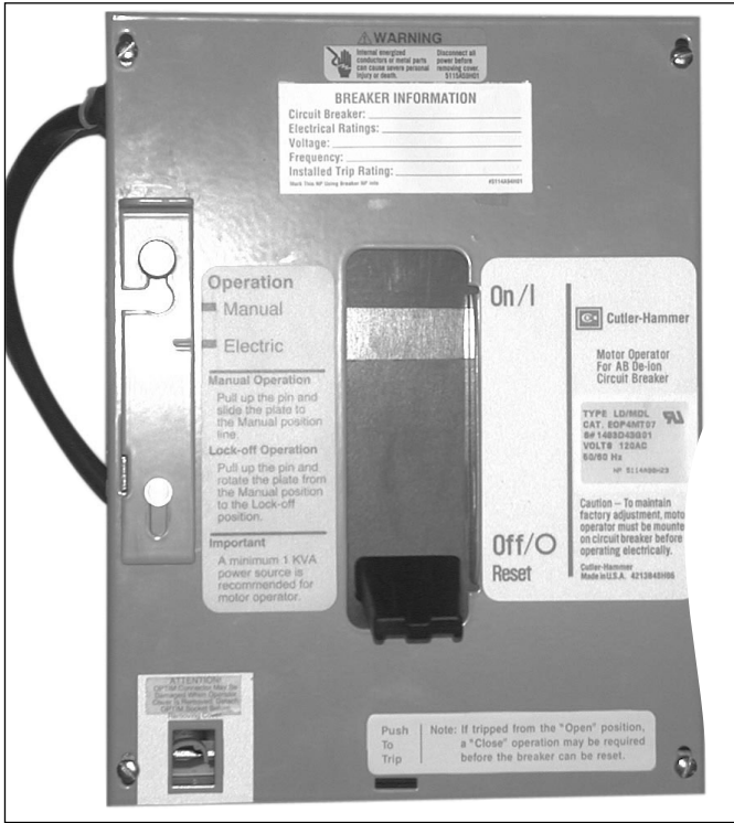
Figure 3-2 Motor Operator in Electrical Position
