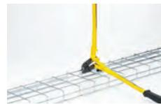
**4** Turn tray open-side down and cut wires from bottom of tray.
