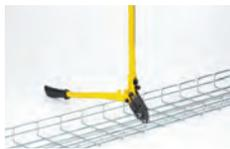
**1** Face tray up. Slide cutter next to vertical wire and cut.
