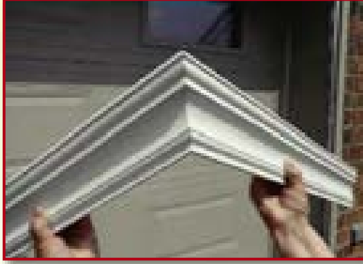
Create perfectly fitting exterior crown molding joints
