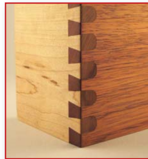
Cuts Through Joints
