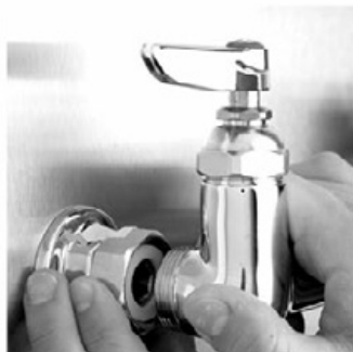
STEP 2 - Remove old control valve by unthreading nut.
