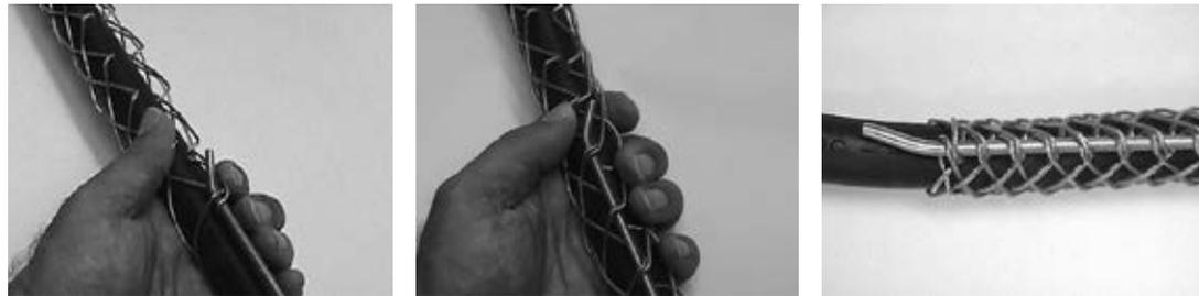
1. Place the grip around the cable. Starting at the eye end, thread the rod through the formed loops with a corkscrew motion. Use the curved leading end of the rod to pull the loops together
