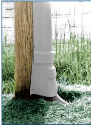
Carlton PV-Mold is a non-metallic pole riser system designed to protect communications or power cable installed on poles.
