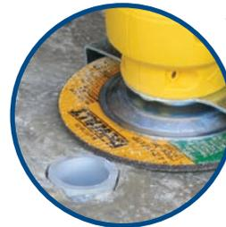
**2.** Insert plug to keep conduit clean/dry through balance of rough-in. Once rough-in is complete, remove plug and continue with step 3.
