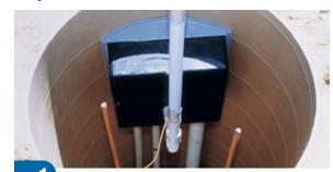
J-Box, with all conduit and fittings placed as desired, is temporarily attached to the concrete form – base and lid inside.
